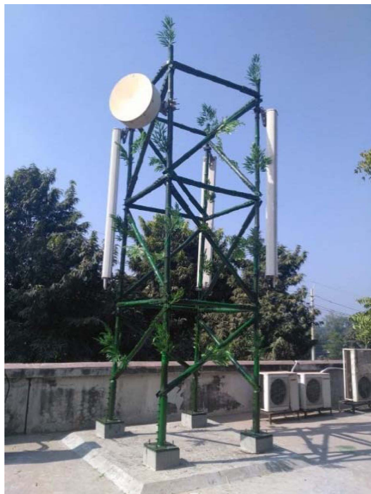
Fig. 1. Bamboo tower placed over rooftop at Dhaka, Bangladesh. (Image by Md. Shahrir Alam.)
