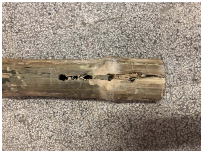
Fig. 10. Tension failure due to tearing through a line along the holes of joints.
